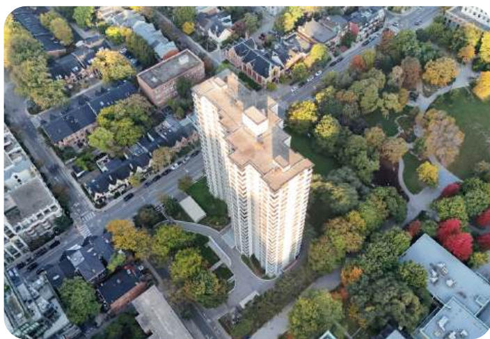
Drone image of subject site, view looking northwest
