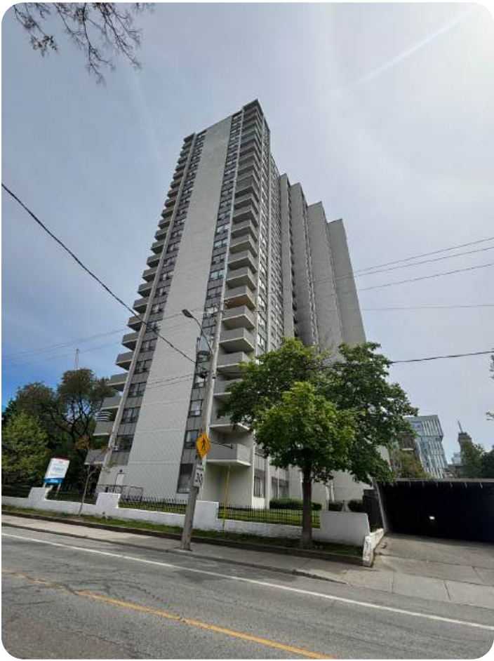
Looking east at the existing building and the access to the existing underground garage
