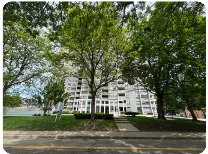
Looking north from Stephanie Street towards the front yard and primary pedestrian access to the existing building
