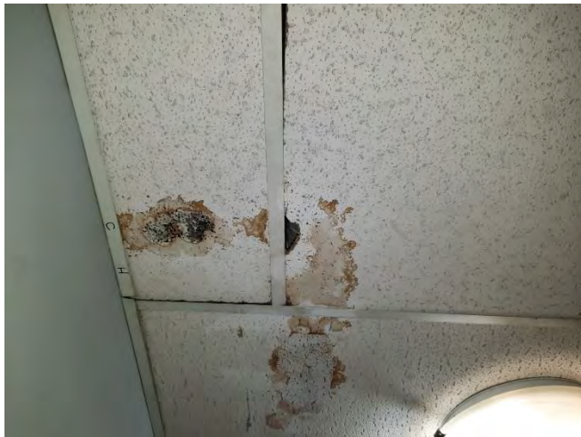
Photo 11: View of one of the suspect mould-impacted ceiling tiles on the 24 th floor of the Subject Building.
