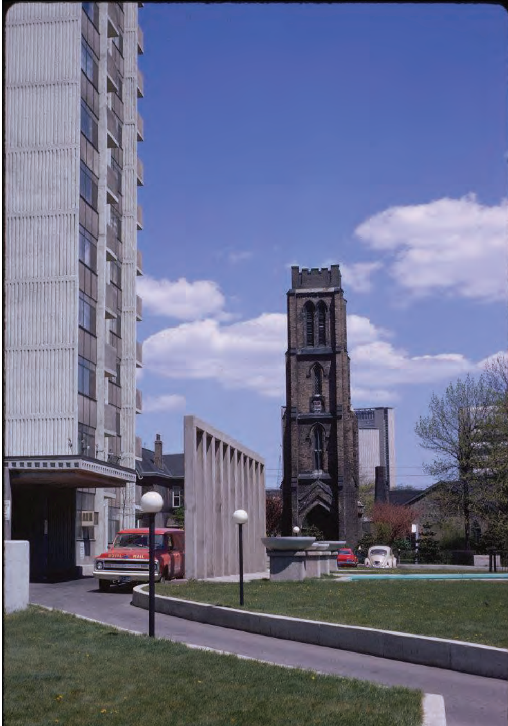
1971 photograph looking east towards the Site and St. George the Martyr Church (City of Toronto Archives).
