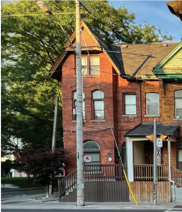
Principal (west) elevation of 39 Beverley Street (ERA, 2025).
