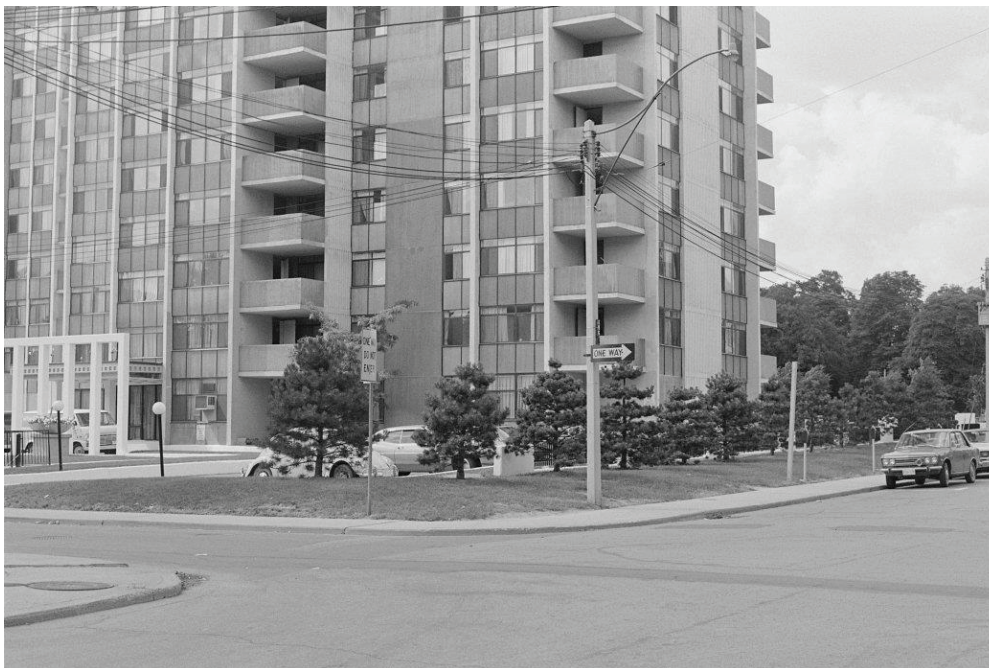
1972 photograph looking northwest from the corner of Stephanie and John Streets towards the Site (City of Toronto Archives).
