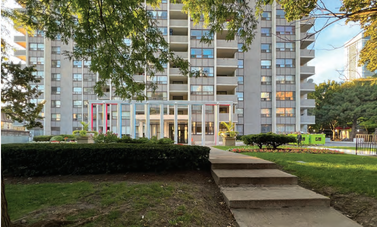
Principal (south) elevation and main entrance to the building on the Site (ERA, 2025).
