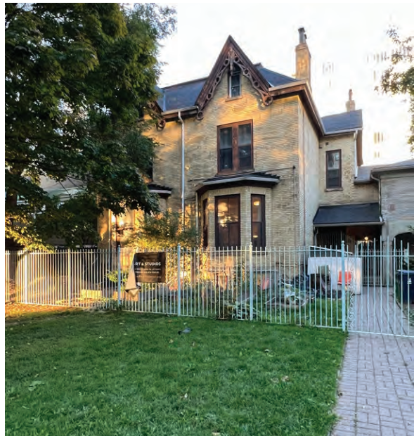
Principal (west) elevation of the rectory (ERA, 2025).
