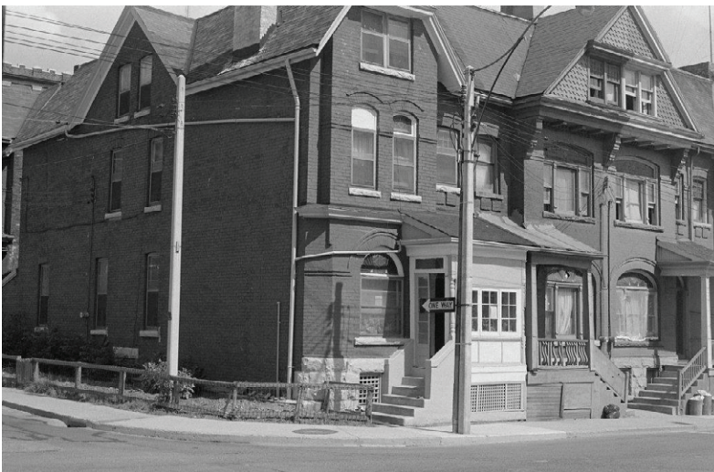
1972 photograph looking southeast from the corner of Beverley and Stephanie Streets towards 39 Beverley Street (City of Toronto Archives).
