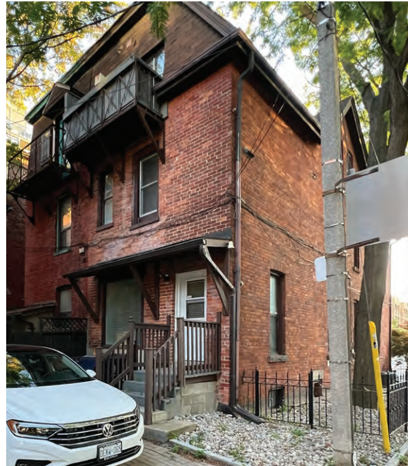
Side (north) and rear (east) elevations of 39 Beverley Street (ERA, 2025).
