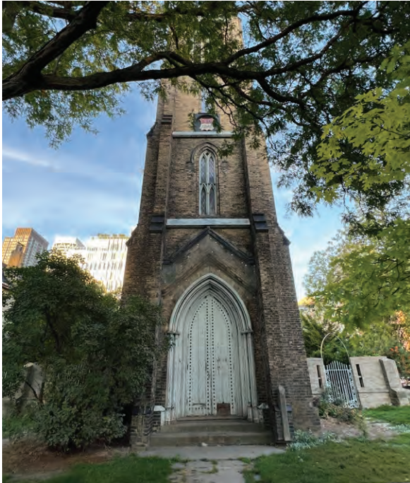
Principal (west) elevation of the bell tower (ERA, 2025).
