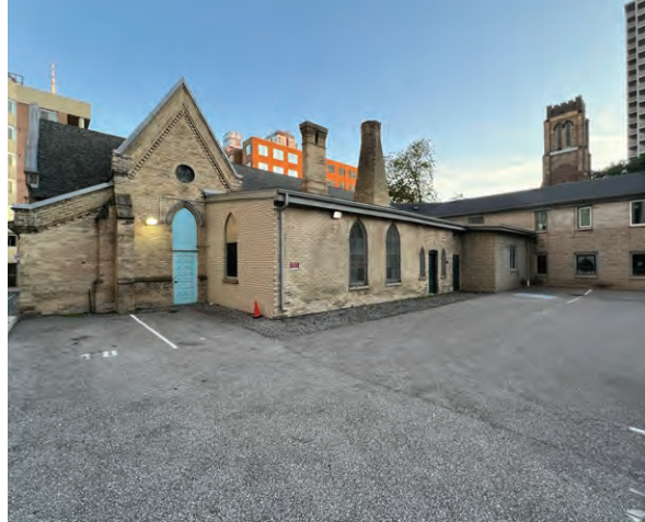
North elevation of the parish hall as seen from across the parking lot at the rear of the property, with a portion of the 1985 addition visible at the right (ERA, 2025).
