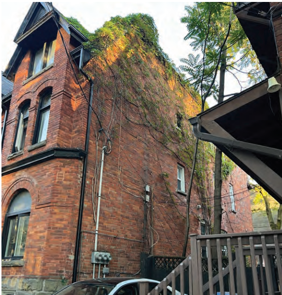
Side (west) elevations of 45-47 Stephanie Street (ERA, 2025).
