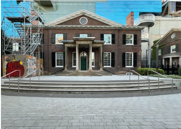
Principal (south) elevation of the Grange (ERA, 2025).
