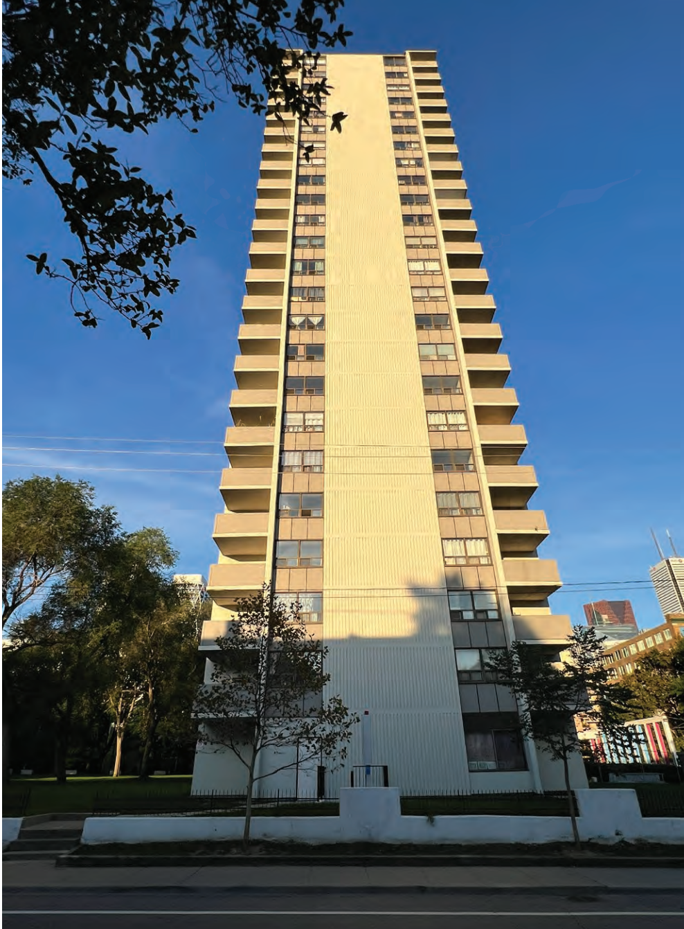
Side (west) elevation (ERA, 2025).
