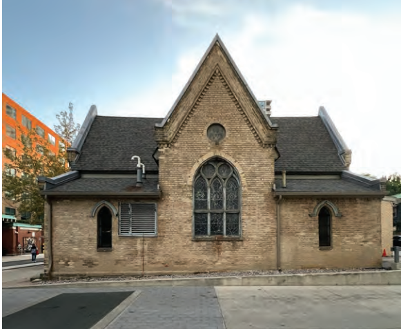
East elevation of the parish hall (ERA, 2025).
