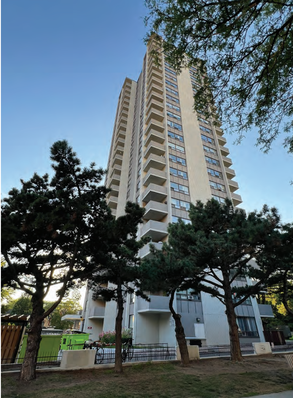
Side (east) elevation (ERA, 2025).
