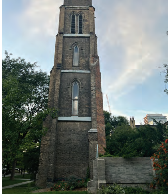
South elevation of the bell tower (ERA, 2025).
