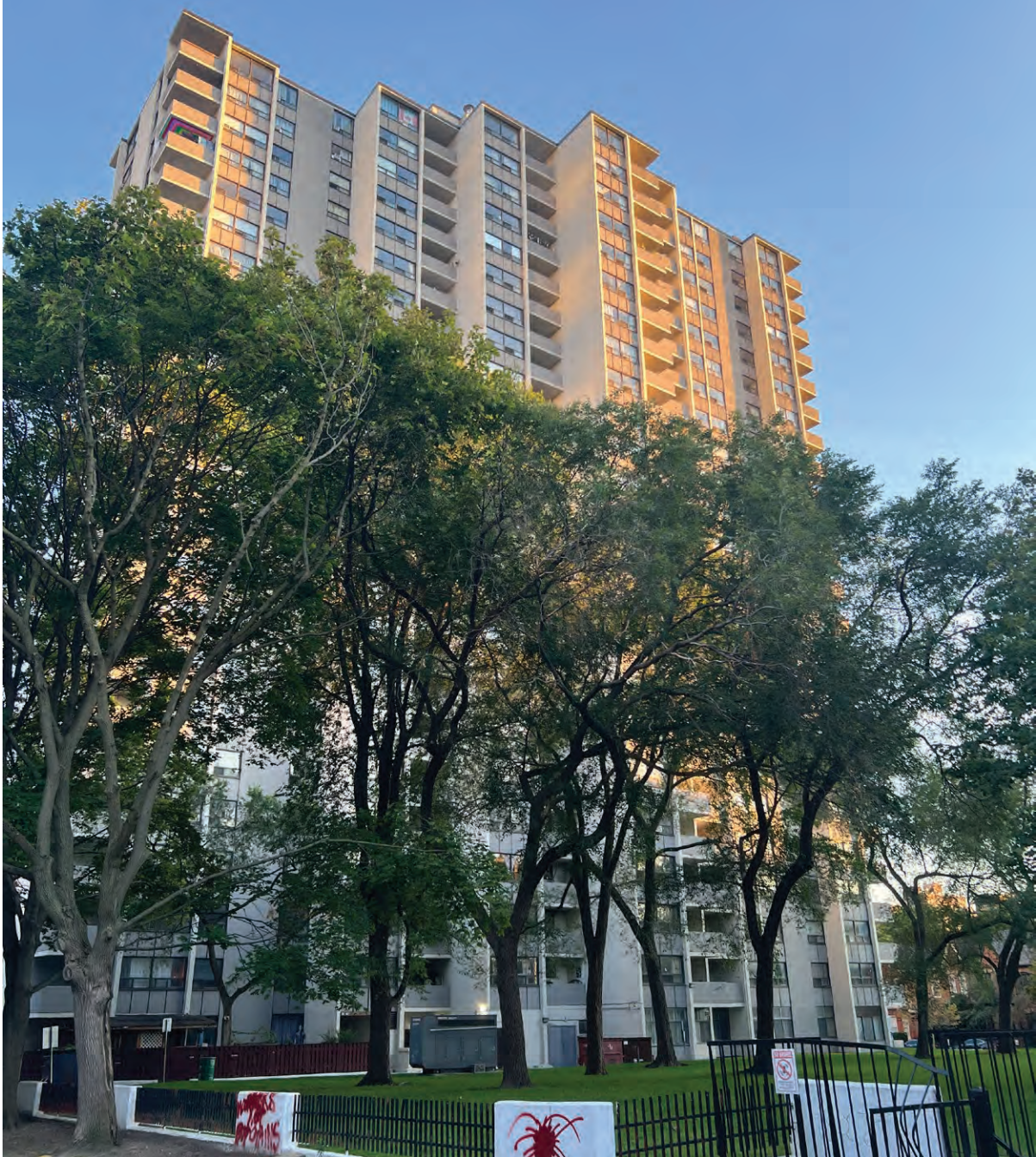
Rear (north) elevation (ERA, 2025).
