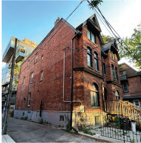
Principal (north) and side (east) elevation of 45-47 Stephanie Street (ERA, 2025).
